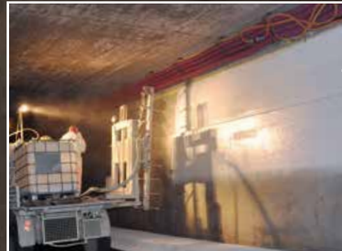
Concrete replacement and surface protection
