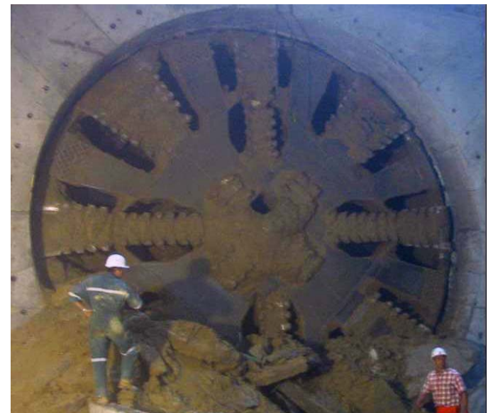
Figure 13: clean cutterhead after breakthrough
