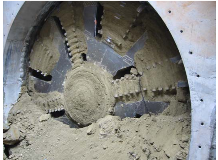
Figure 2: clay clogging in Toulouse Line B Lot 2
