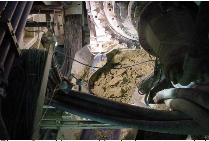
Figure 5: problems working in dry compressed air mode
