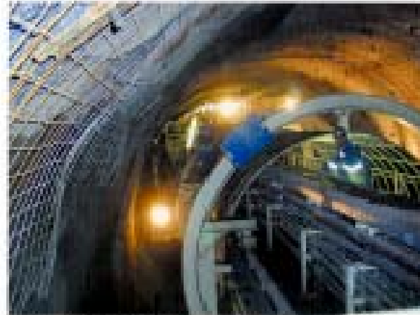
■ Circular beam structure for wet-mix sprayed concrete application on the TBM back-up. High capacity and the best concrete quality.
