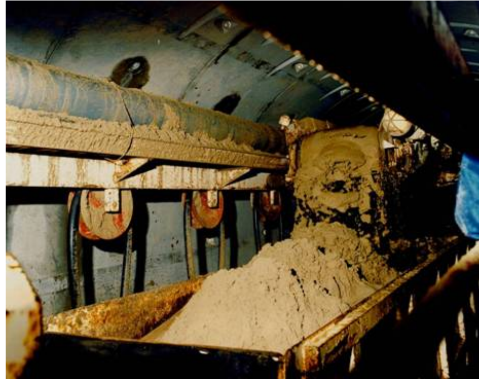
2.5 bar sea water pressure use of foam & polymer
