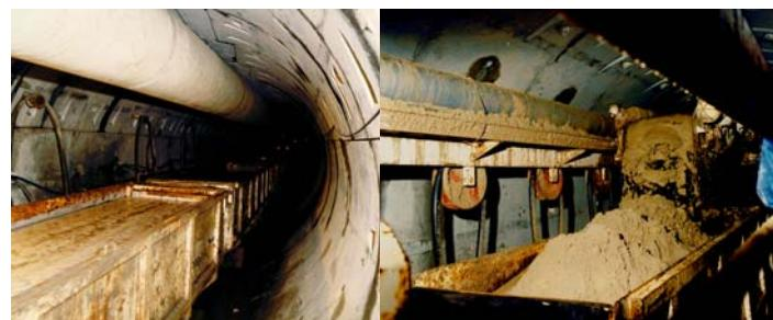
polymers: left side only foam used, right side dry sand excavation by using foams in combination with polymers.
