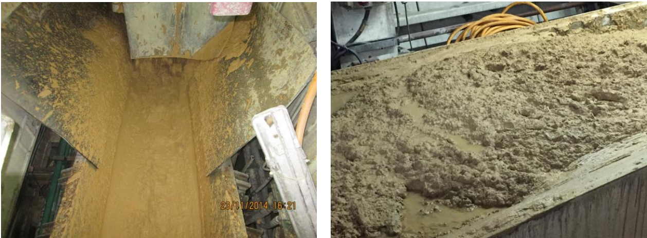
Fig. 7 Excavated soil: coming out of the screw conveyor, muck car
