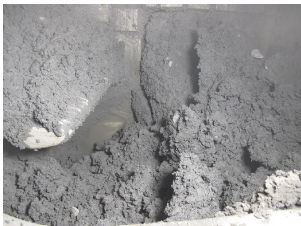
Picture 11: Well conditioned soil inside the TBM working chamber
