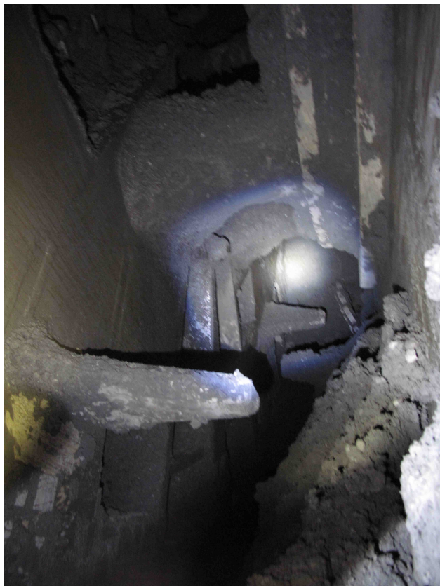
Picture 12: clean chamber after finishing EPB mode
