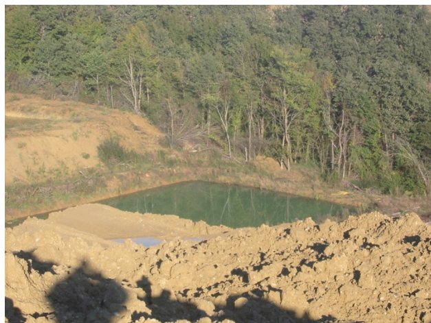
Figure 5. Land modelling with excavated soil & surface water retention basin at Metro Toulouse project, France.
