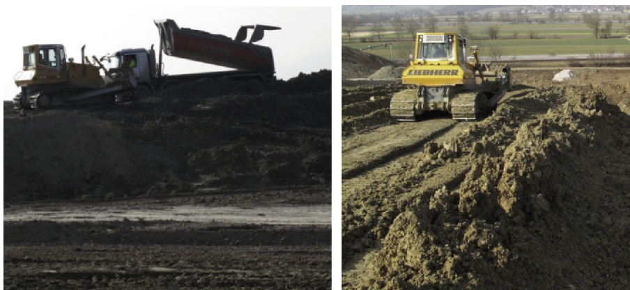
Fig. 9. Disposal of conditioned soil with favorable consistency.
